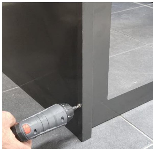
4. Join front panel to side panel with 2x M6 screws, repeating for other side
