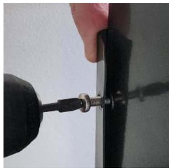
7. Connect side panel to wall strips on both sides using M6 screws
