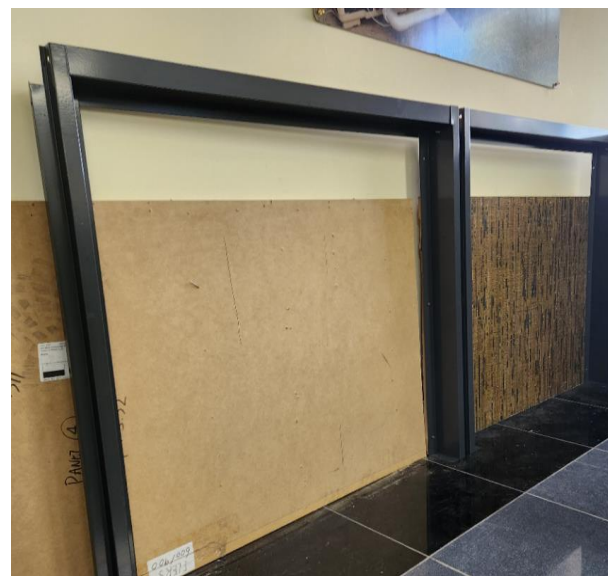
6. Ensure both sets of wall strips and bridges are square & secured to wall
