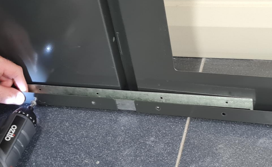
8. Secure bottom channel to front panels using 4x tap screws, as per step 2
