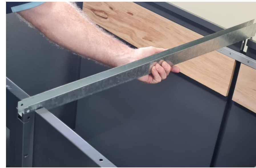
13. Position join channel between front and rear panels
