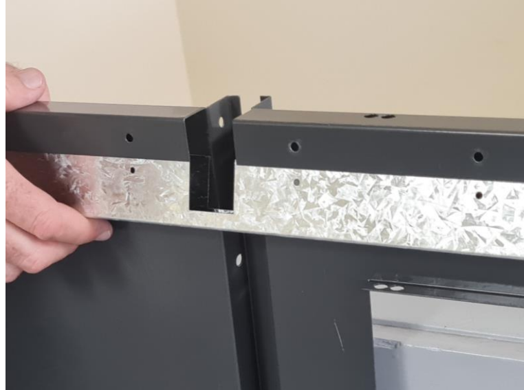
9. Slide top support channel into top of both front panels
