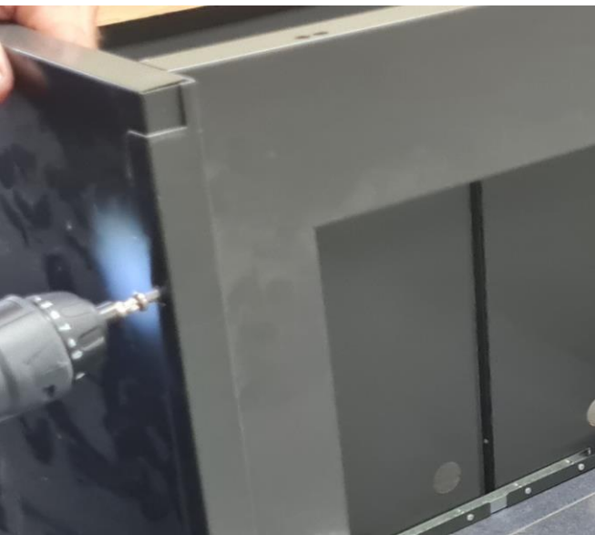
11. Join side to front panel with 2x M6 screws, repeating for other side
