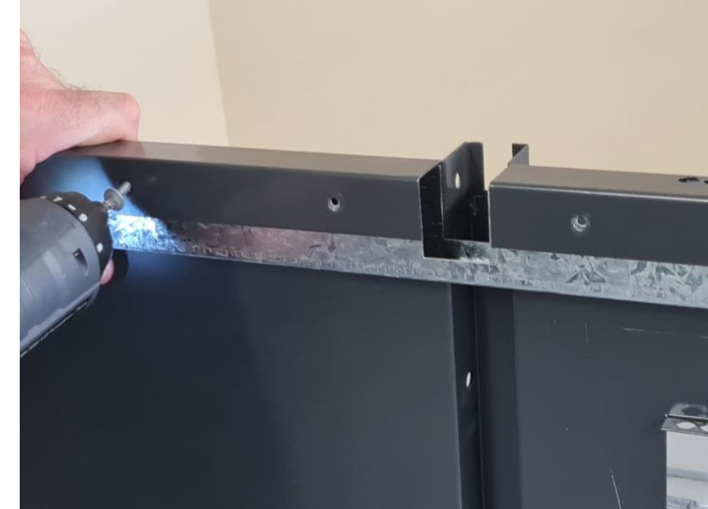
10. Secure top channel to both front panels using 4 x tap screws
