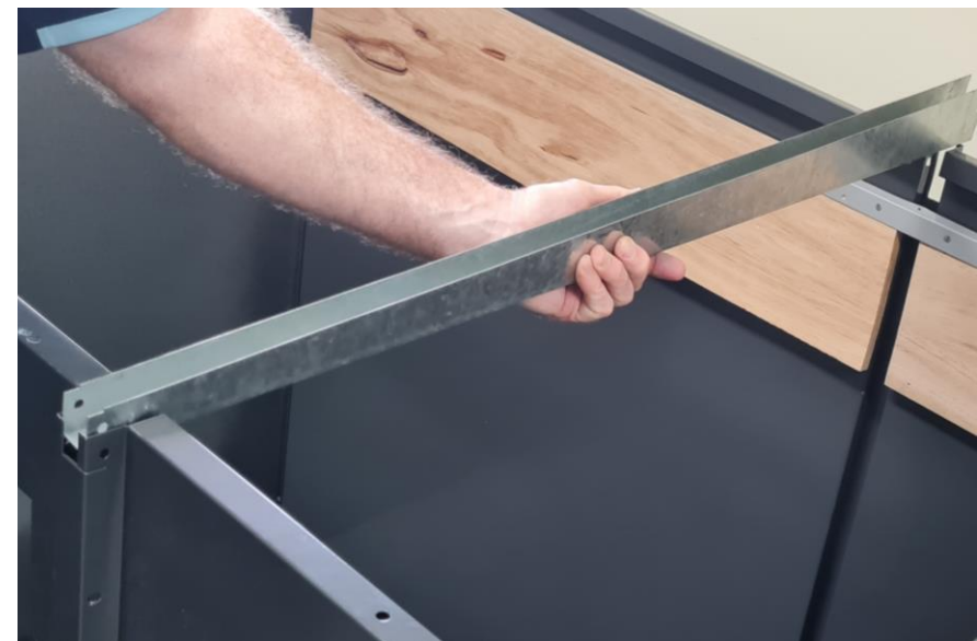
14. Position join channel between front and rear panels
