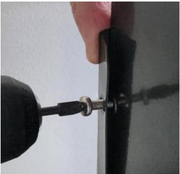
**5. Connect side panel to wall strips on both sides using M6 screws**
