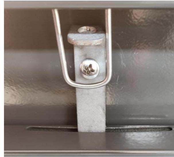
**16. Insert latch into door to hold in place**
