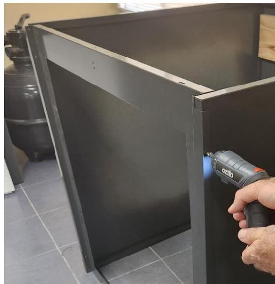
**7. Join front panel to side panel with 2x M6 screws, repeating for other side**
